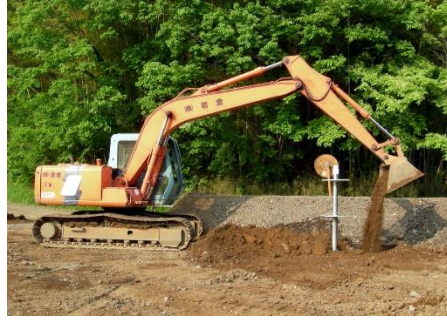
Figure 2. If the ground is hard due to gravel or industrial waste, a power shovel or other excavating equipment is needed to dig a deep hole.
